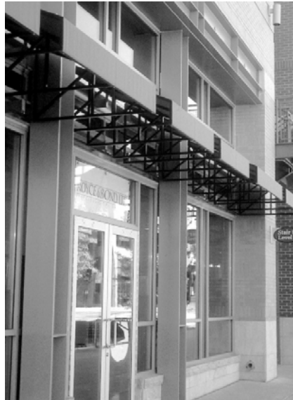
A new commercial storefront should incorporate traditional storefront elements such as display windows, transoms, and a recessed entry.
