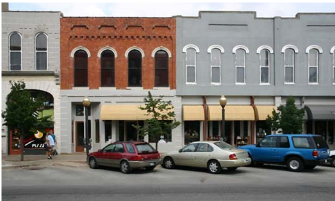
Patterns of fenestration and detailing should be retained on upper stories.
