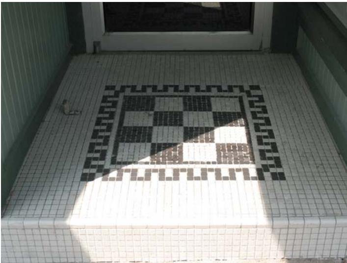
Material details such as these inlaid tiles should be retained.
