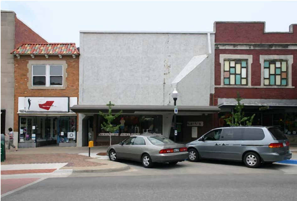
It is inappropriate to remove or cover upper story architectural features.
