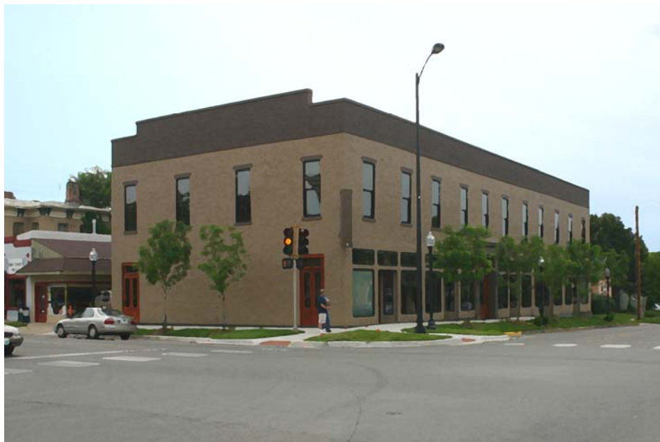
By design, secondary facades should be related to, but not in competition with, primary elevations. In this example the secondary facade shows some compositional balance, but has too little articulation and too low a percentage of window at the street level.
