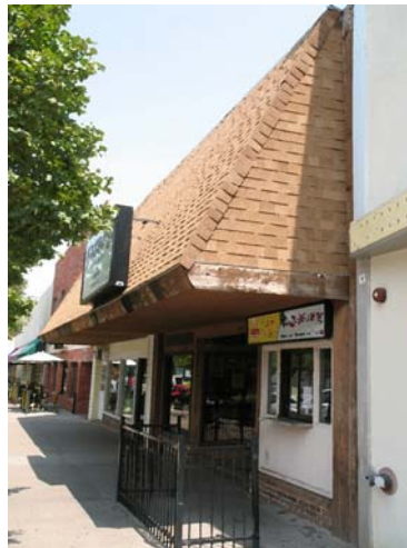
'Permanent' awnings clad in asphalt or wooden shingles, trellis-work, or other materials that are more typically found in residential areas, are not
