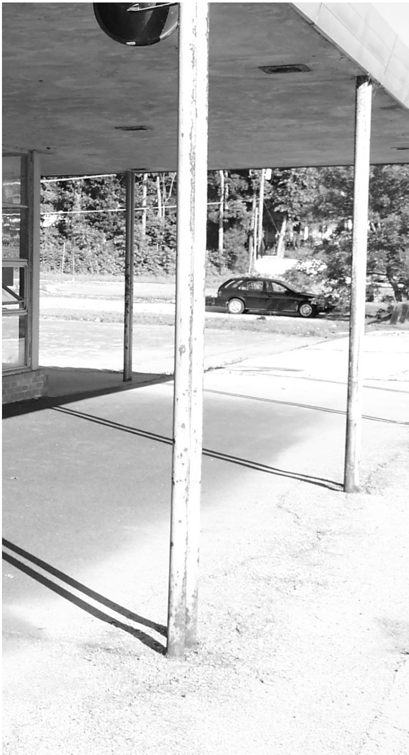
The Platform of the Lawrence Santa Fe Depot is elevated to eliminate the need for stools when boarding passenger cars.
