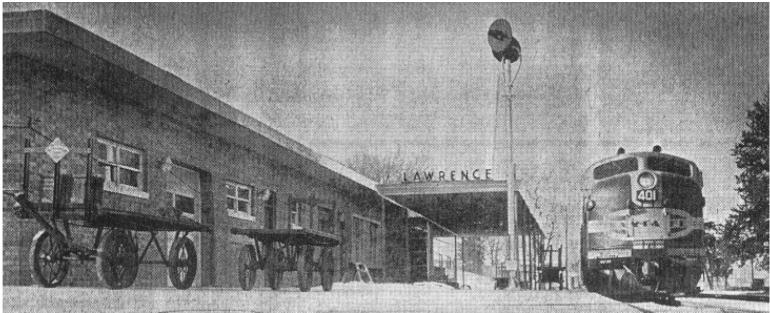
"There isn't a more modern station in the system!" -Ellis . P. Addy, Lawrence Santa Fe agent, 1956
