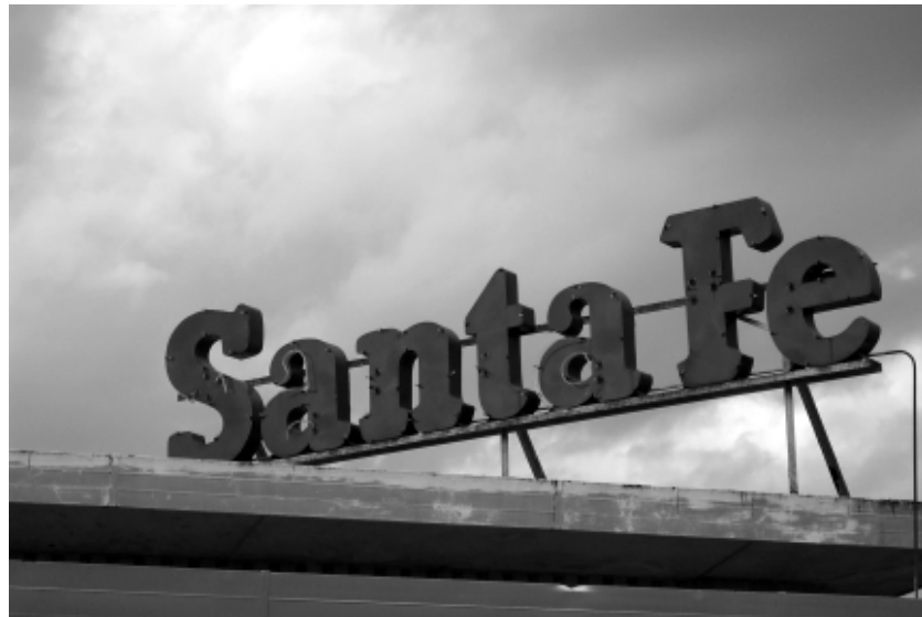
A neon sign , positioned to be recognized from downtown, once illuminated the Santa Fe above the main entrance to the depot
