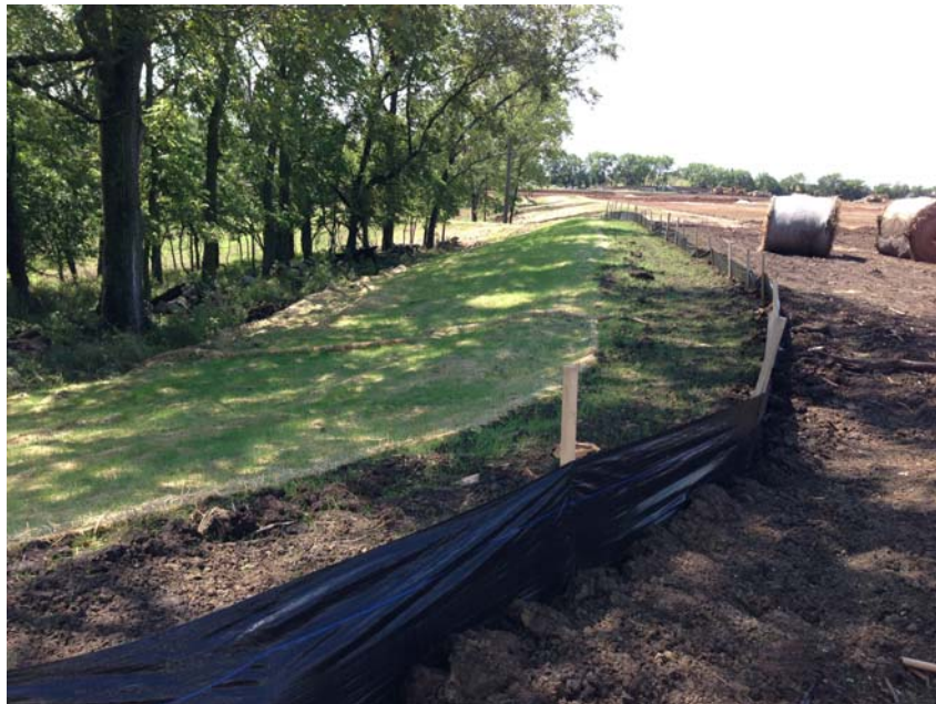
Seeding established outside of silt fence
