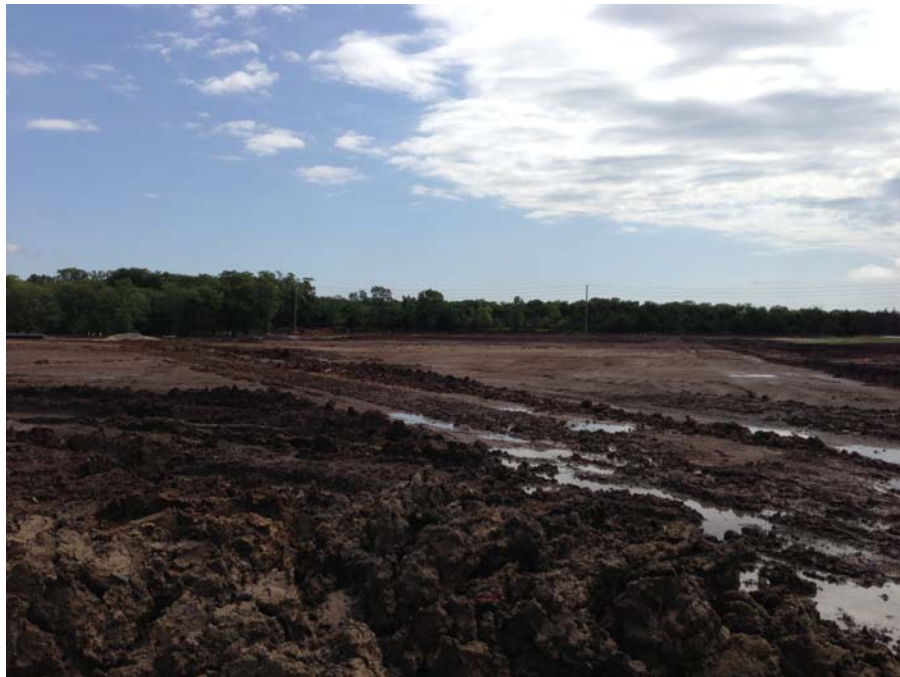
Southern parking lots graded (looking east)
