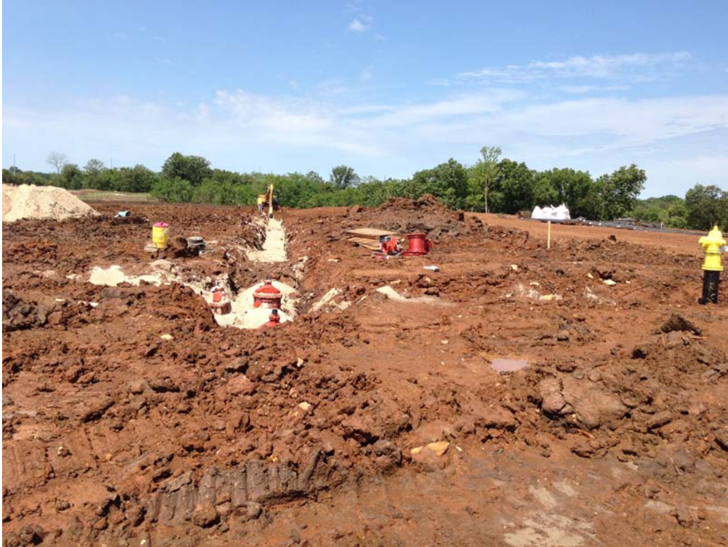
Waterline being installed south of rec building
