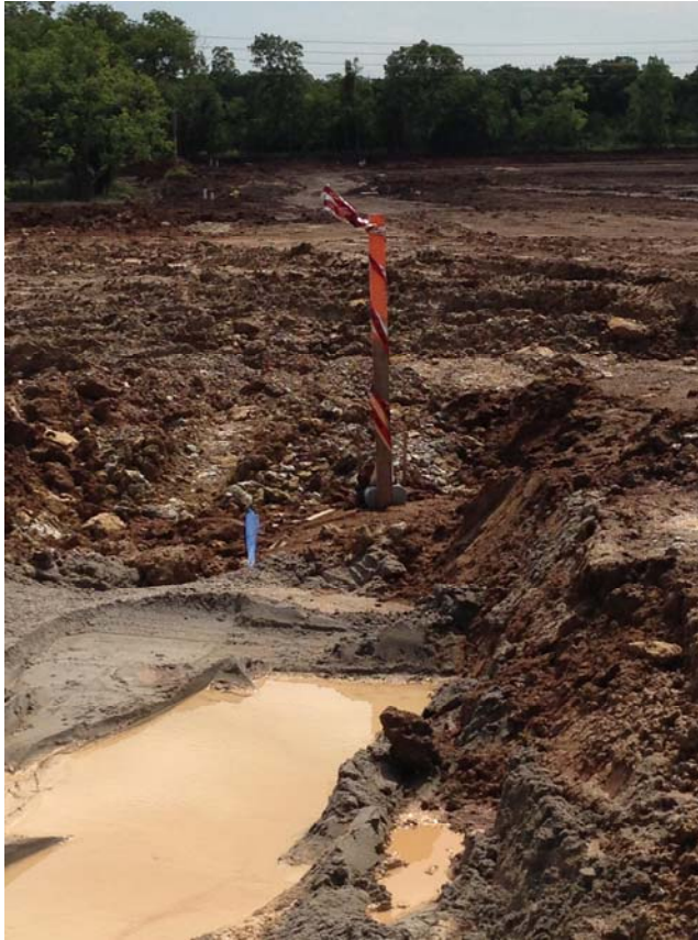
Dual 4" Conduits installed with waterline (capped at base of stake)
