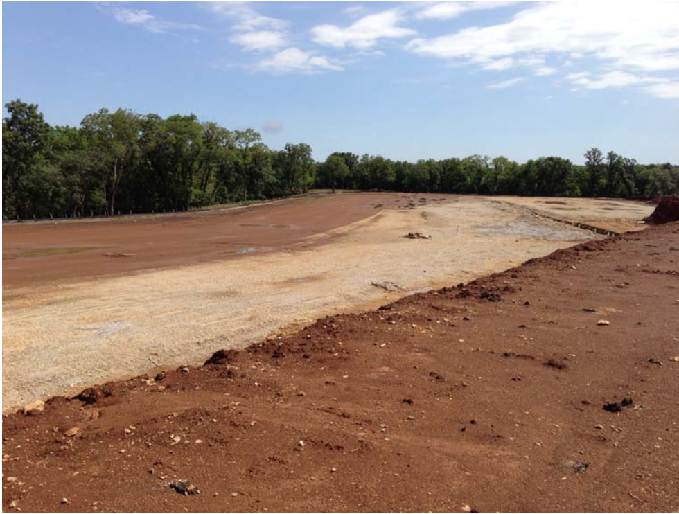
Rec Center pad (looking east)
