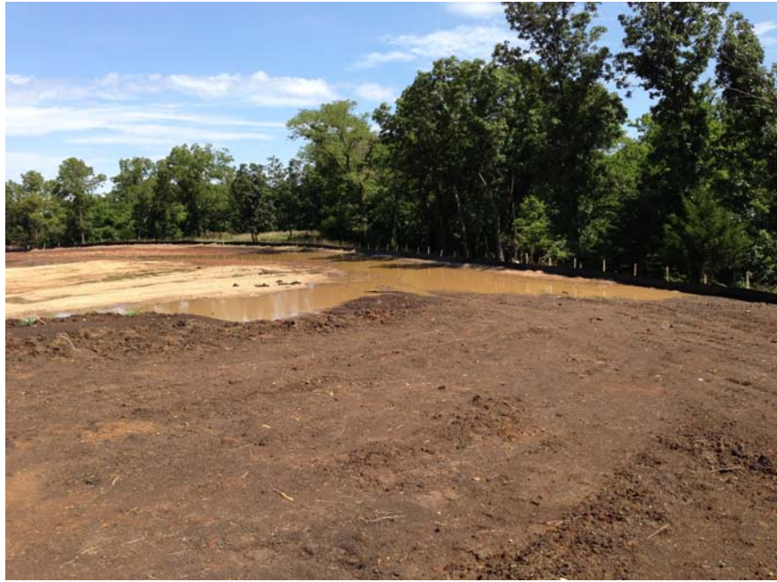
Silt fence retaining sediment on north end of silt
