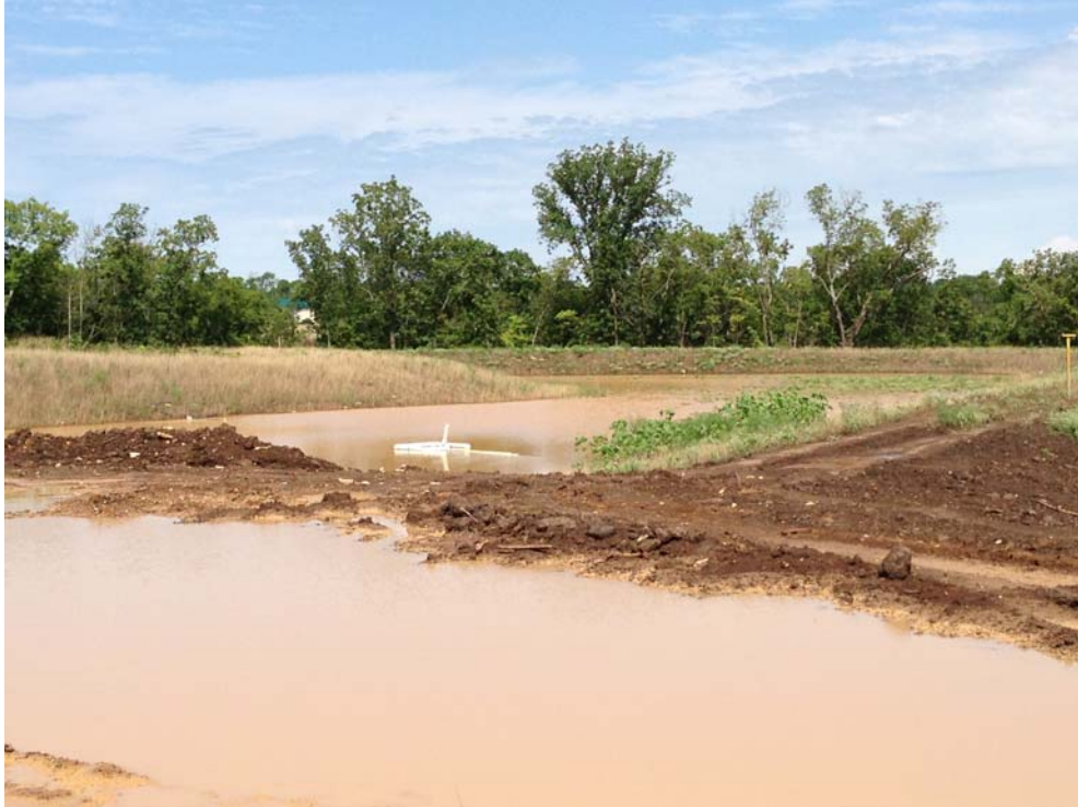
North Detention Pond
