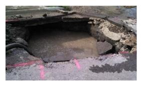
The water main leak caused a large hole, 20 ft  $\times$  10 ft on East 19<sup>th</sup> Street and Bullene.
