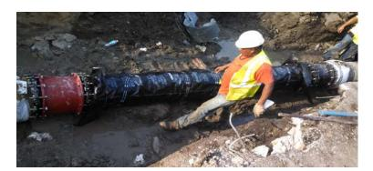
New repair kit and pipe installed
