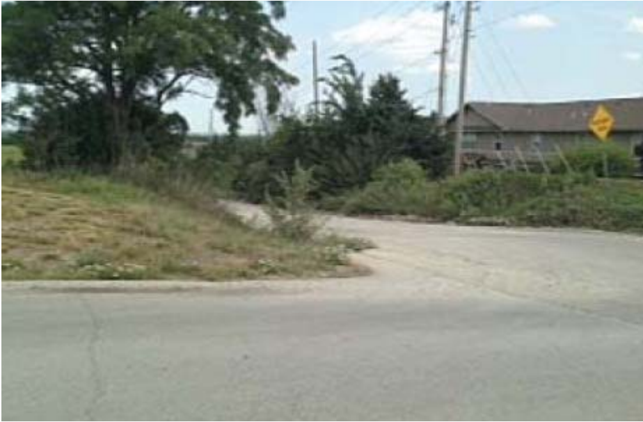
Eastbound looking North
