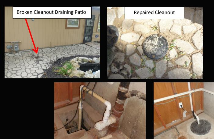
Sump Pump Connected to Sanitary Sewer
