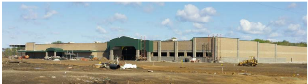
Photo of Menards Store under construction.
