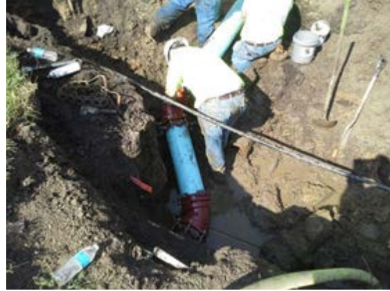
Forrest Avenue Water Main Replacement
