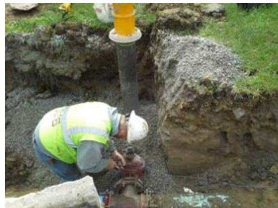
Haskell Avenue Water Main Replacement
