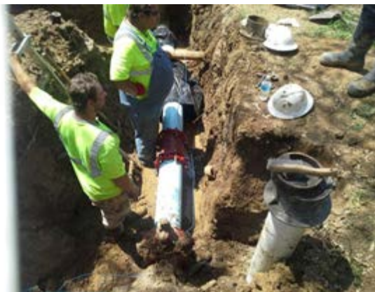
Maple Lane Water Main Replacement
