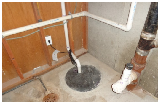
New Sump Pump Discharging Outside
