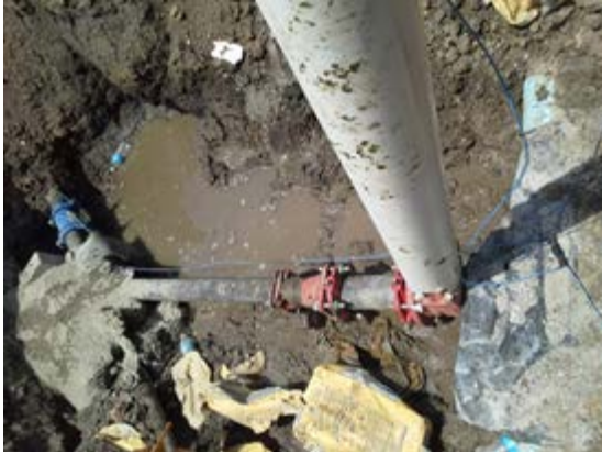
New Jersey Street Water Main Replacement
