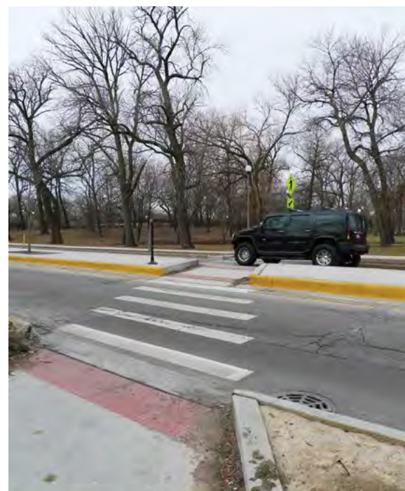
Figure 9. Pedestrian Refuge Island on a Road Diet Corridor in Chicago Photo Credit: Stacey Meekins
