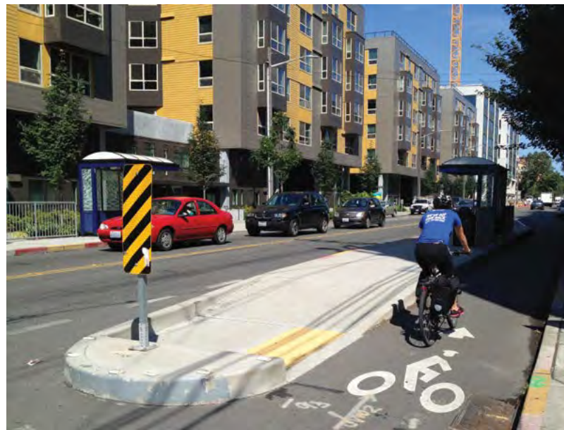
Figure 13. Bus Loading Zone in Seattle, Washington Photo Credit: City of Seattle
