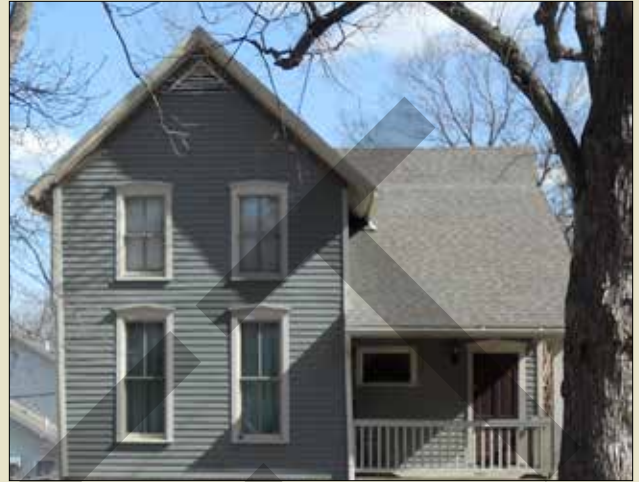
These fiberglass shingles are approximately the scale of the original roofing shingles.
