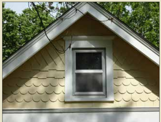
Wood shingles used on gable end.
