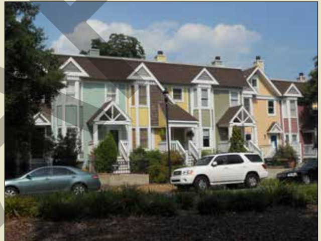
Multi-dwelling structure has individual front doors.
