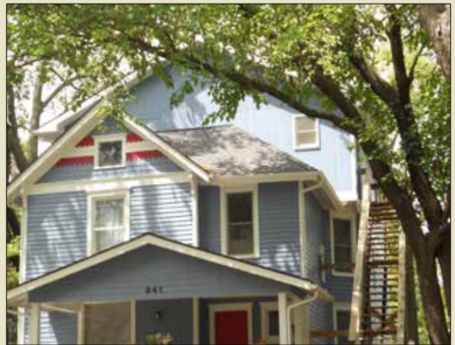
Here an unacceptable addition overwhelms the original building.
