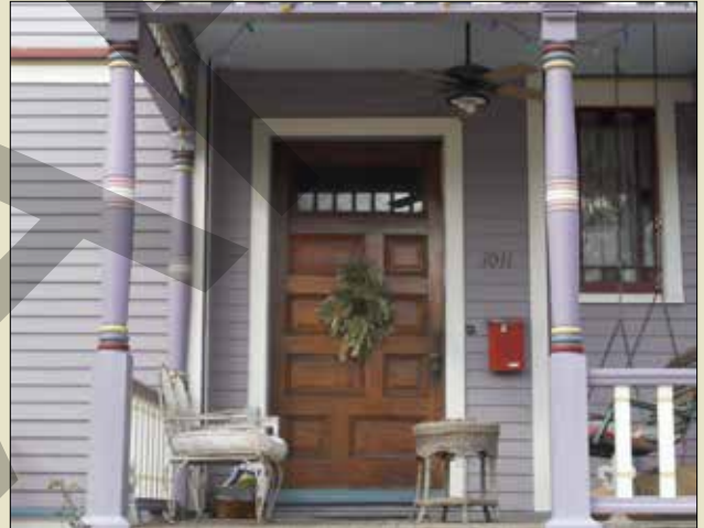
Retain original doors, door surrounds, side lights and transoms, like this example.
