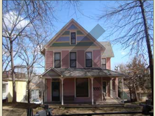
Retain the appearance, character and arrangement of architectural features, such as in this example.
