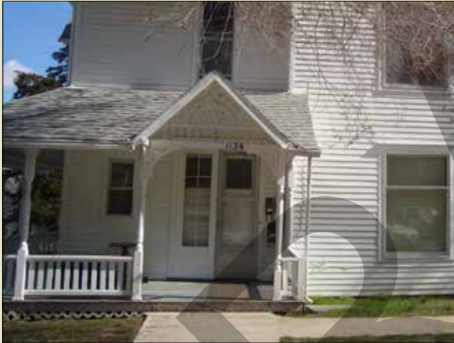
Balustrades are composed of a series of balusters that collectively make a screen that is slightly more opaque than transparent.
