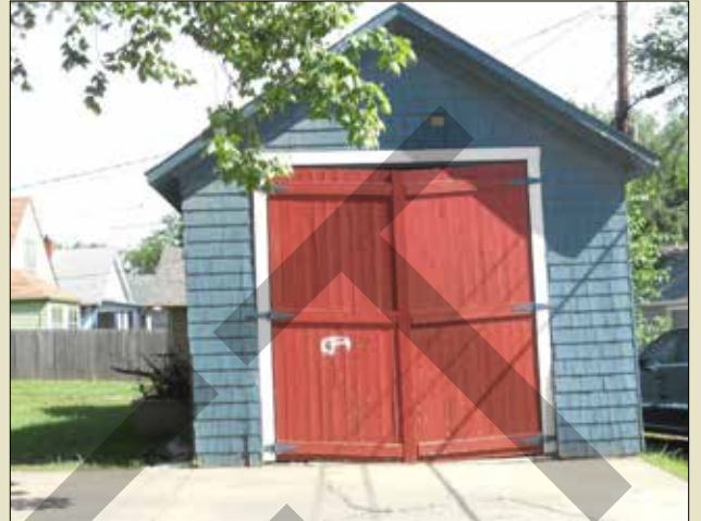
Garage doors should reflect the style of the main house and character of the district.
