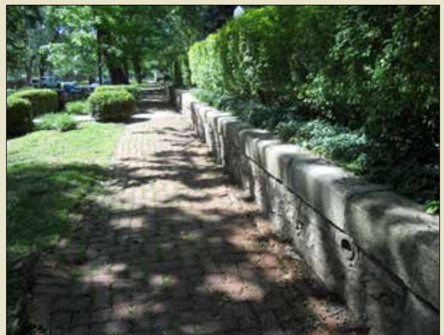
Retaining walls were traditionally low and made of native stone.
