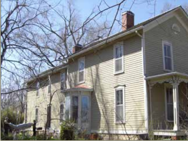
A good example of how a slight recess helps distinguish the addition from the original.
