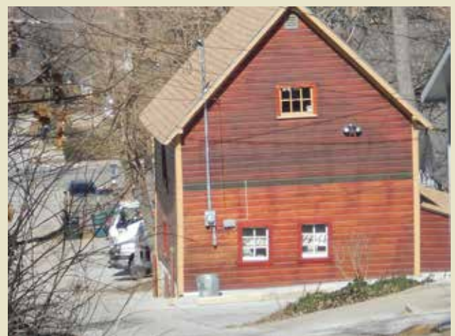
Historic accessory structures like this carriage house are important to the character of a neighborhood.
