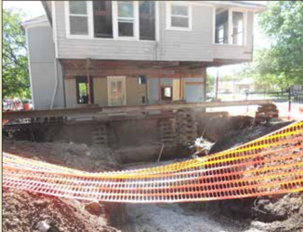
Rehabilitation of an existing structure.
