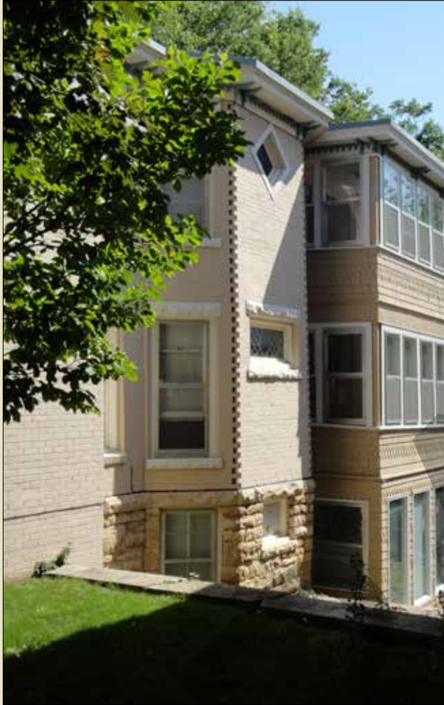
A good example of how character-defining features on the front of the building shall be preserved.
