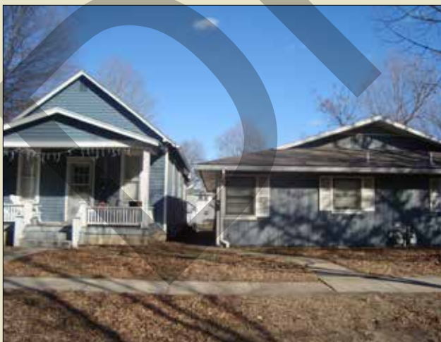
A newer structure that has been built to the current side yard setback increases density.
