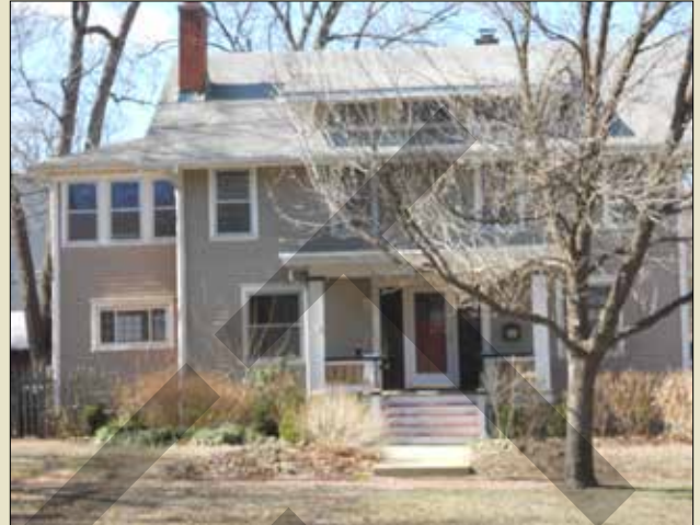
A acceptable example of how additions should be subordinate to the primary structure.
