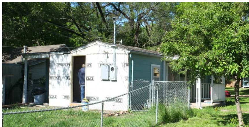
Area of Damage
