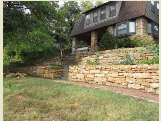
A good example of a stepped retaining wall in Oread.
