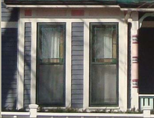
Window placement and patterns are character defining features.
