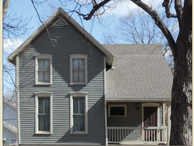
These fiberglass shingles are approximately the scale of the original roofing shingles.
