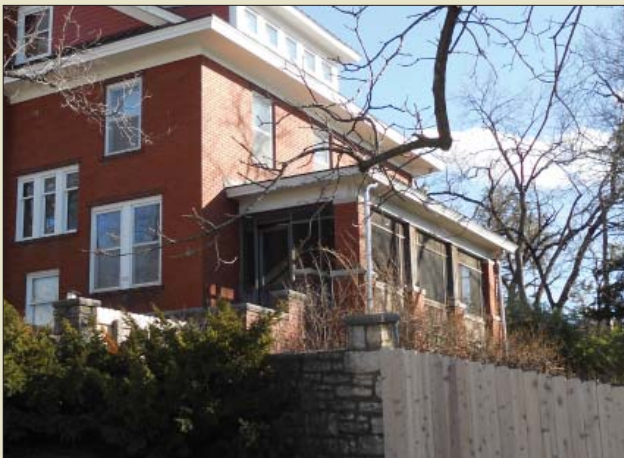
If a front porch is screened, it shall be constructed so that the primary architecture elements, such as columns and balustrades are readily visible from the street.
