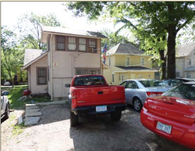
Parking lots have crept up to the rear doors.
