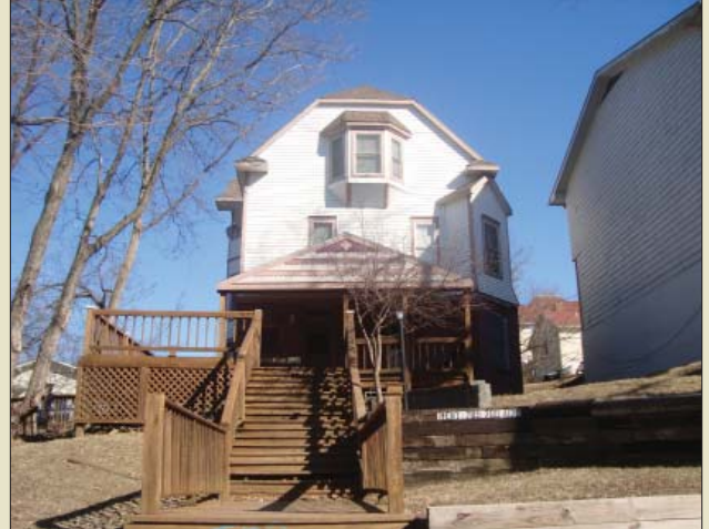
An unacceptable example showing why all decks should be on the rear of the structure and not visible from the front yard.
