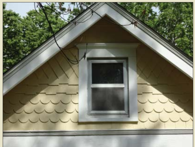
Wood shingles used on gable end.
