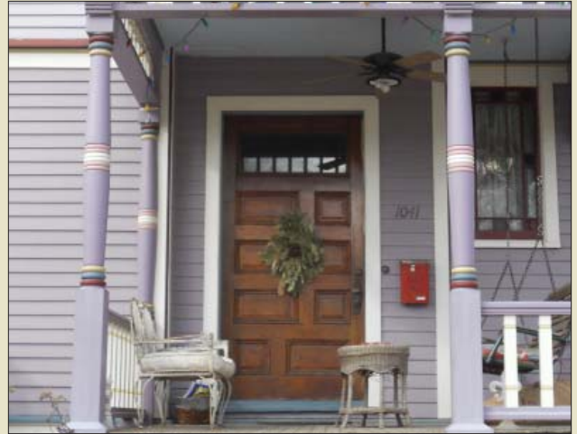
Retain original doors, door surrounds, side lights and transoms, like this example.
