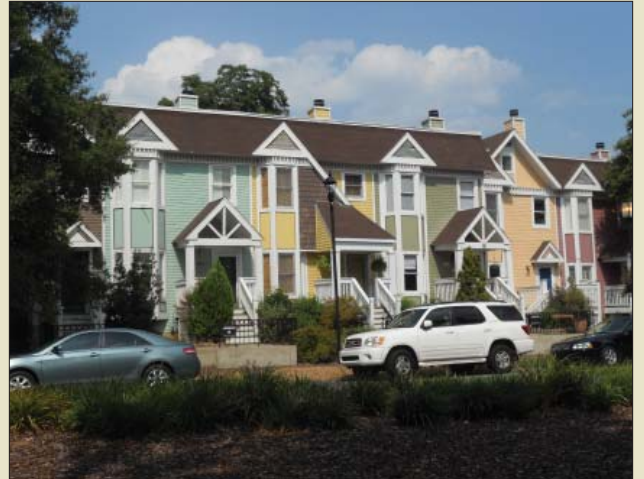
Multi-dwelling structure has individual front doors.
