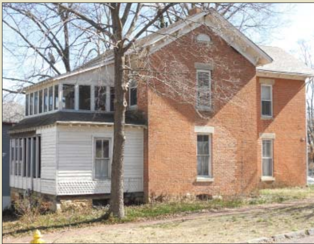
An unacceptable addition at the rear of the property.
