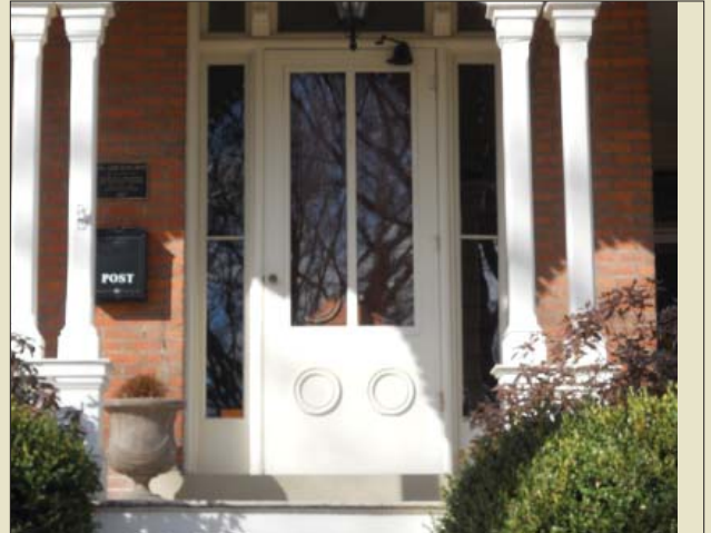
Location, style and size of doors are important character defining features.
