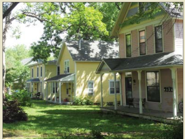
Development of the lot and site - relationship of primary building to street and neighbors.
