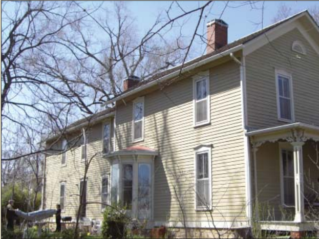
A good example of how a slight recess helps distinguish the addition from the original.
