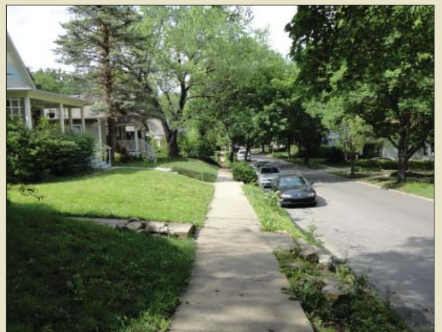
Yards are often graded down to the sidewalk without the use of retaining walls.
