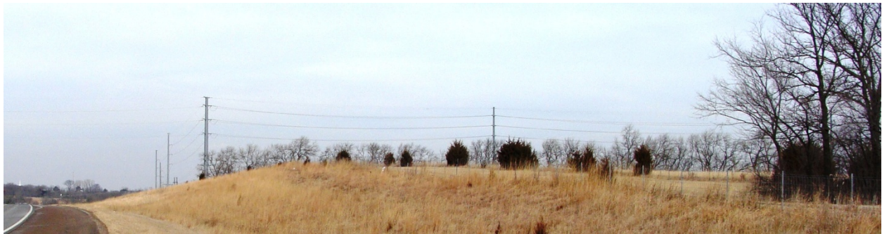
Figure 7: Existing Overhead power lines presently on-site, facing north.
