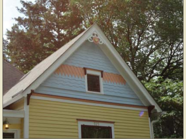
Primary roof form shall either be a gable end, cross gable, hipped, pyramidal, or gambrel.
