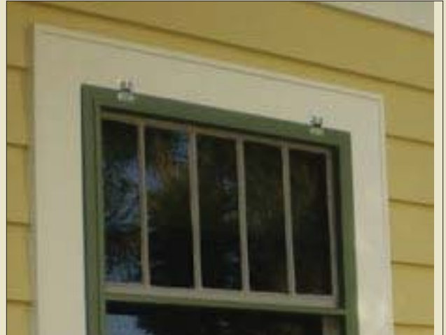
A good example of painted, wooden storm windows that are appropriate for this application.
