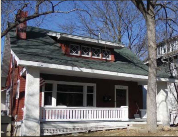
Retain original porch details such as the balustrade, columns, and porch skirting.
