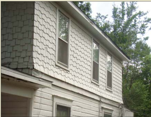
Wood siding and wood shingles are common wall cladding.
