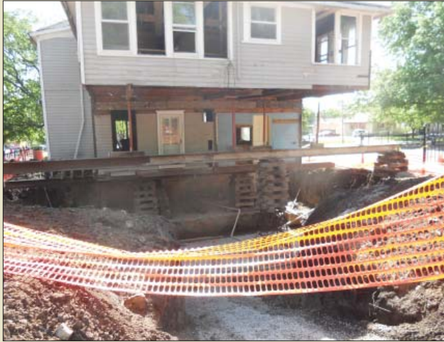
Rehabilitation of an existing structure.
