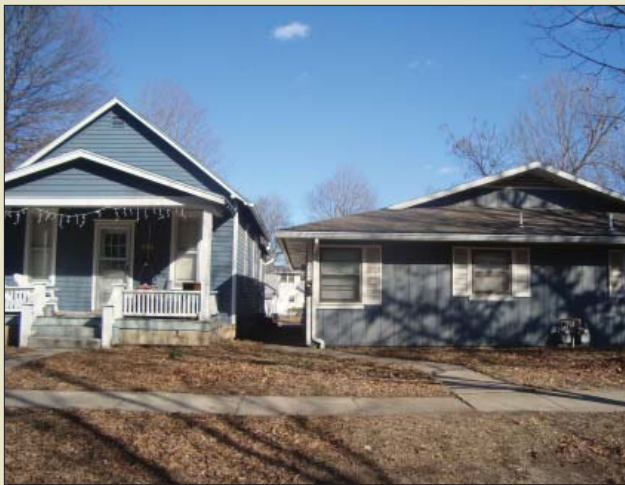
A newer structure that has been built to the current side yard setback increases density.
