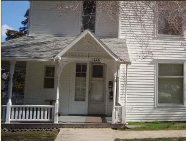
Balustrades are composed of a series of balusters that collectively make a screen that is slightly more opaque than transparent.
