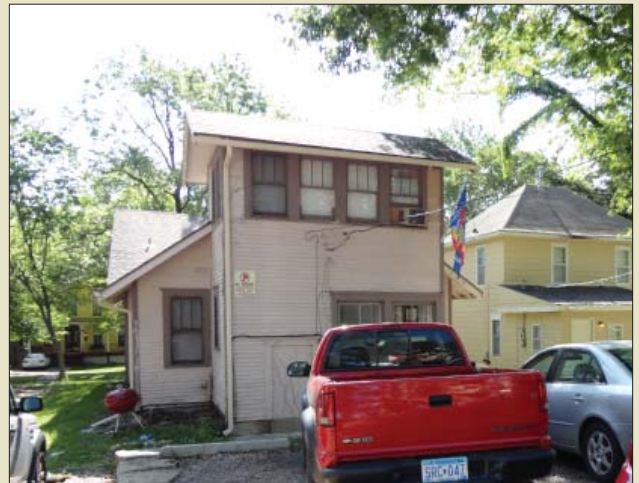
Inappropriate alterations and additions can be removed.
