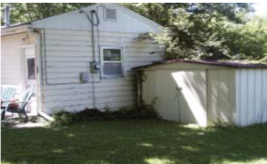
Before Comprehensive Rehab
