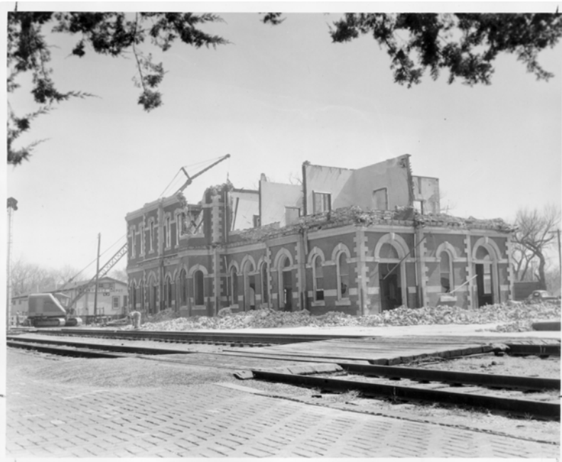
File Name : RH PH 18 A 68, Demolishing Santa Fe Depot, May 1955.jp
