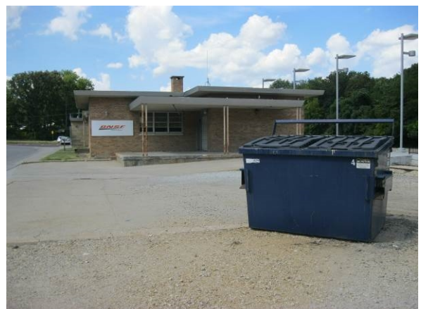
Photo #6 Image of dumpster located on the southeastern portion of site.
