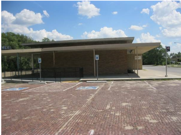
Photo #1 Facing southeast, image of the northwest side of structure.
