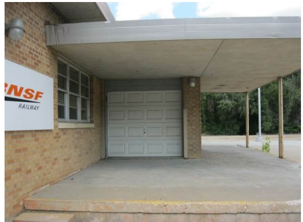
Photo #4 Image of the southeast portion of the structure.
