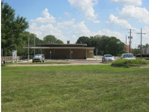
Photo #7 Facing southeast, from the northwest side of site.
