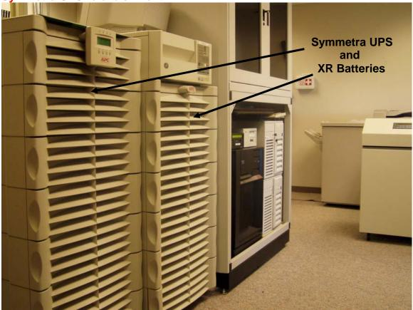
Included in the 2005 budget request is a capital outlay request to recondition the uninterruptible power system (UPS) in the City Hall computer room. Reconditioning involves replacement of the 14 batteries and various system components to extend the system warranty for an additional two years.
