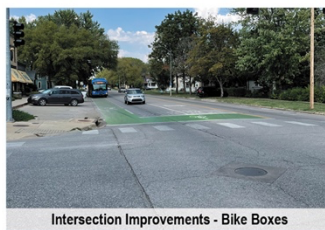
Intersection Improvements - Bike Boxes
