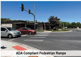
ADA Compliant Pedestrian Ramps
