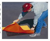
and the wastewater can be collected for proper disposal. Storm drain covers/mats are frequently used along with a vacuum device (e.g. sump pump, wet/dry vacuum, and vacuum pump) that diverts wastewater into the sanitary sewer system.
