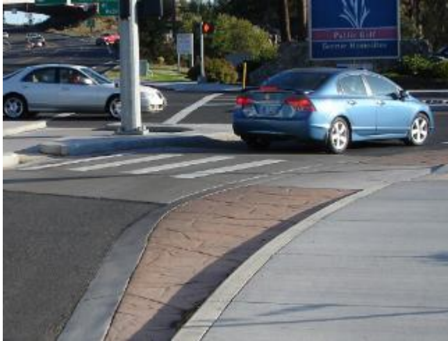
Figure 6-7: Mountable Apron and Raised Crosswalk (Source: Google)
