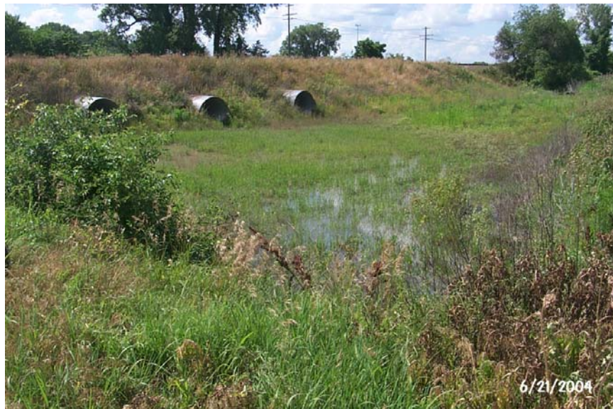
3-108" CMP under RR tracks, west of 24/40 intersection
