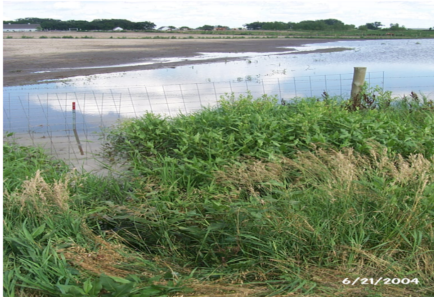
Ponding downstream of 1400/1900 intersection, south of Midland
