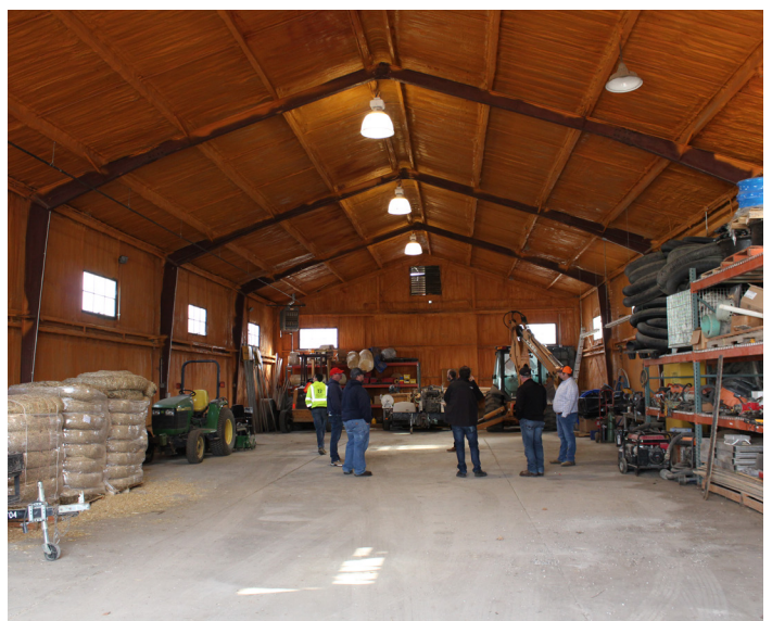
Concrete floor, pre-engineered steel structure, pendant lights, overall good condition
