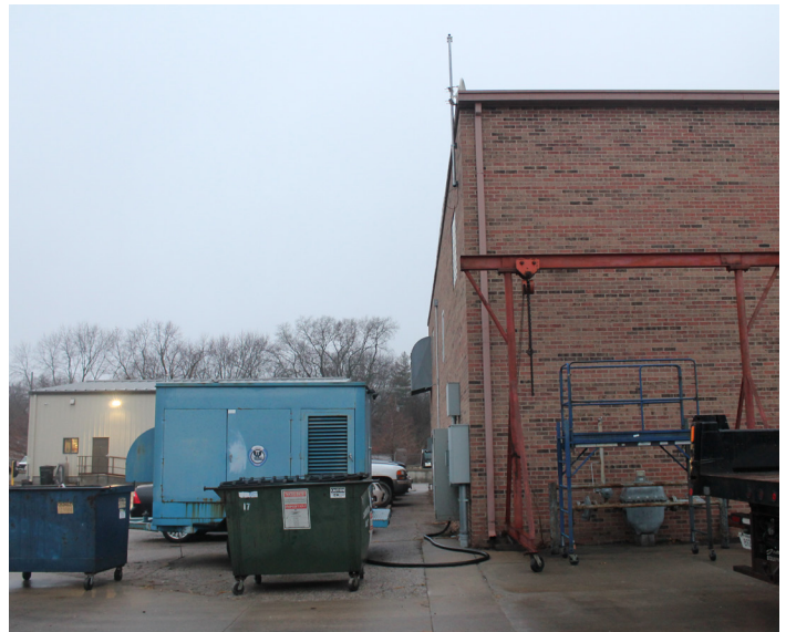
Exterior - good condition
