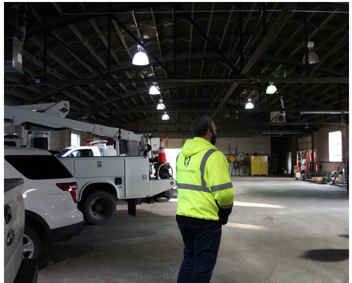
Concrete floor, CMU walls, exposed structure
