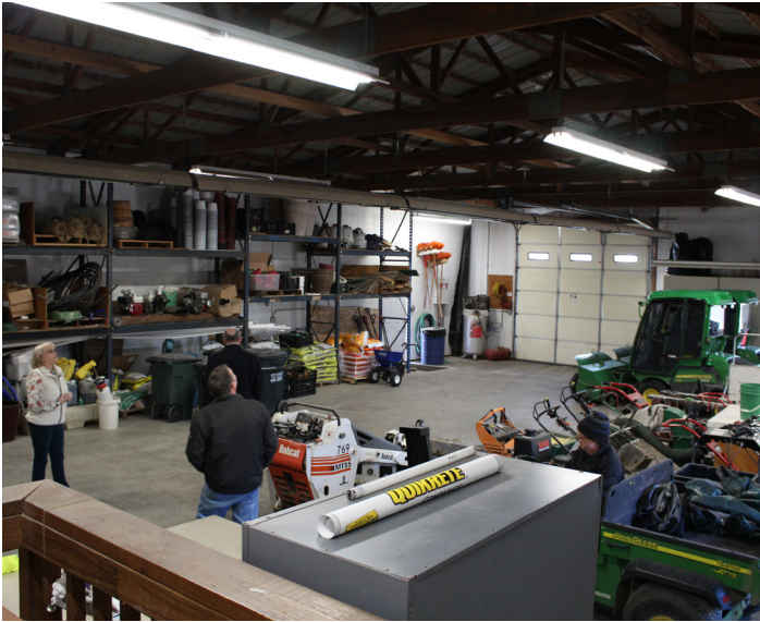
Concrete floor, pre-engineered metal structure, good condition
