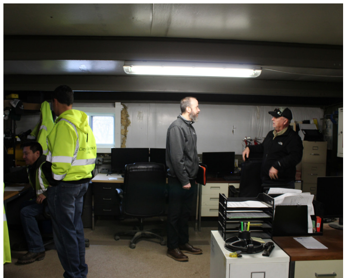
Concrete floor, steel structure, bag insulation, surface mounted fixtures, overall poor condition
