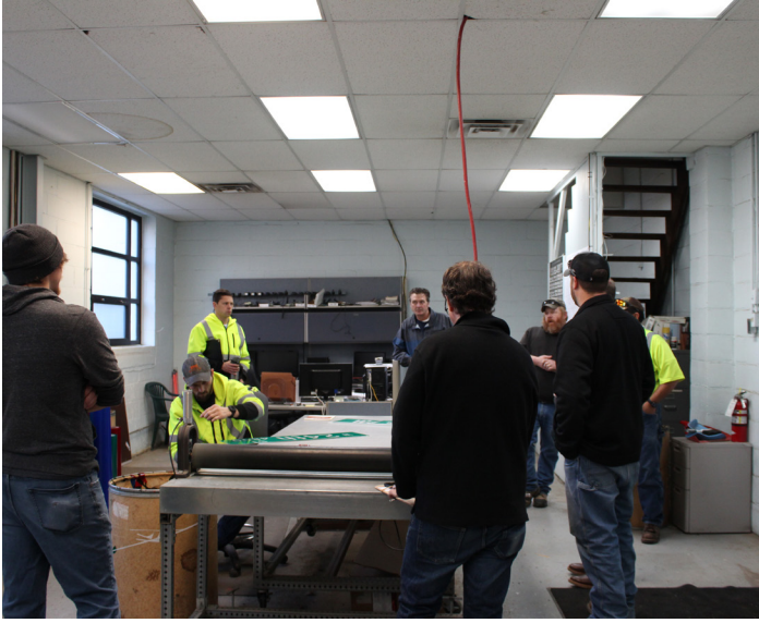
Concrete floor, painted CMU walls, ACT ceiling, fair condition
