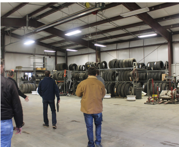
Concrete floor, pre-engineered steel structure; good condition
