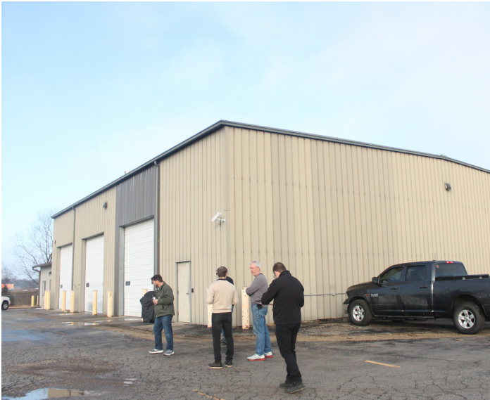
Exterior - fair condition
