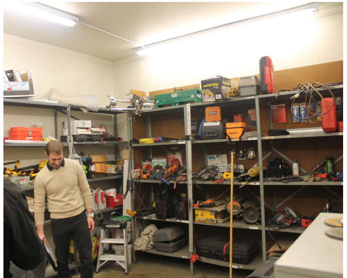
Concrete floor, painted gypsum board walls and ceiling, surface mounted lights
