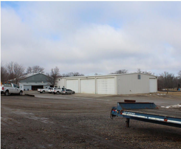
Exterior - fair condition
