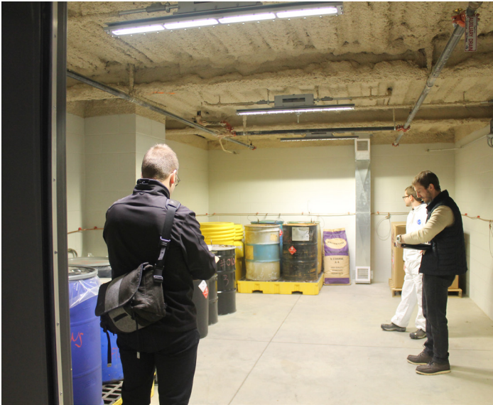
Concrete floor, painted CMU walls, good condition
