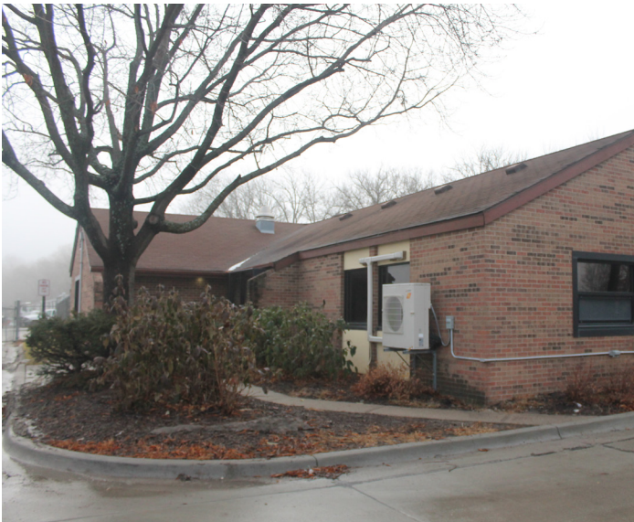
Exterior - good condition
