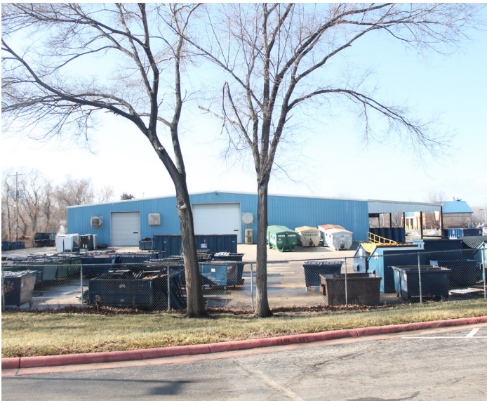
Solid Waste - exterior, good condition
