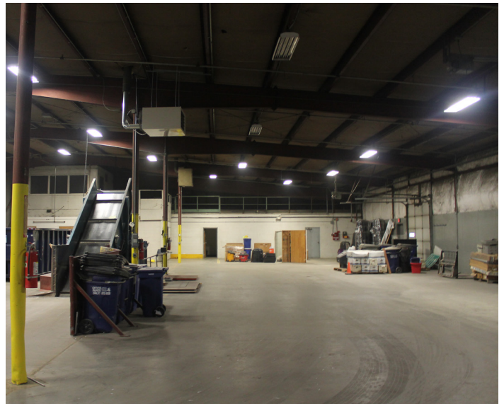
Concrete floor, pre-engineered steel structure, good condition
