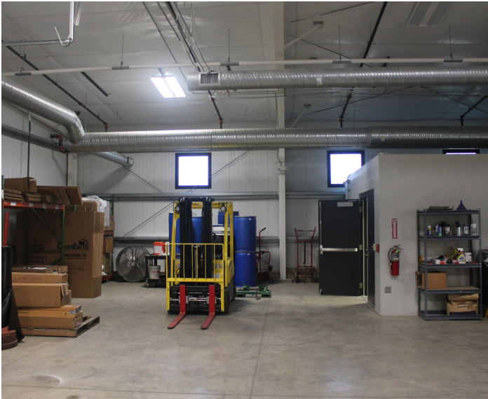
Concrete floor, pre-engineered steel structure, bag insulation, good condition
