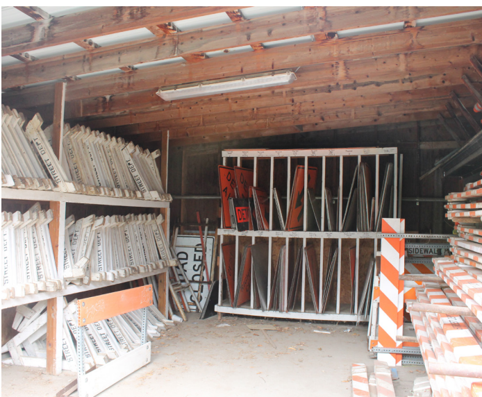
Learn-to structure, surface mounted fixture, good condition
