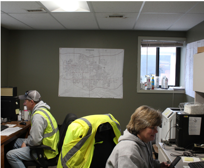
Concrete floor, painted gypsum board walls, ACT ceiling, fair condition
