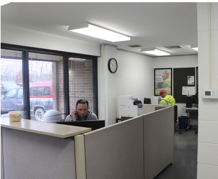
Linoleum flooring, painted CMU walls, gypsum board ceiling, surface mounted fixtures
