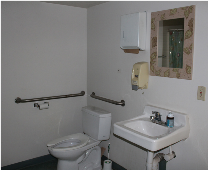
ADA accessible restroom, gypsum board walls
