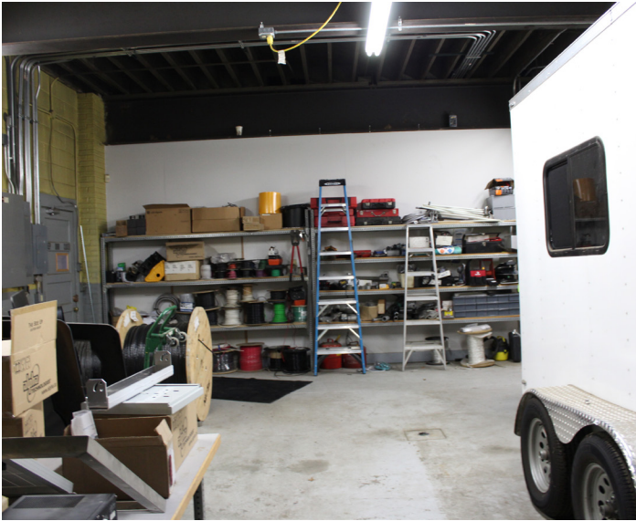
Concrete floor, painted CMU and gypsum board walls, fair condition
