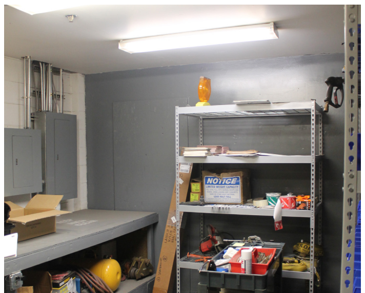
Concrete floor, painted CMU walls, gypsum board ceiling, surface mounted fixtures
