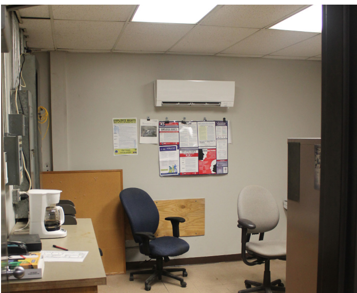
Linoleum floor, 2'x4' ACT ceiling, poor condition
