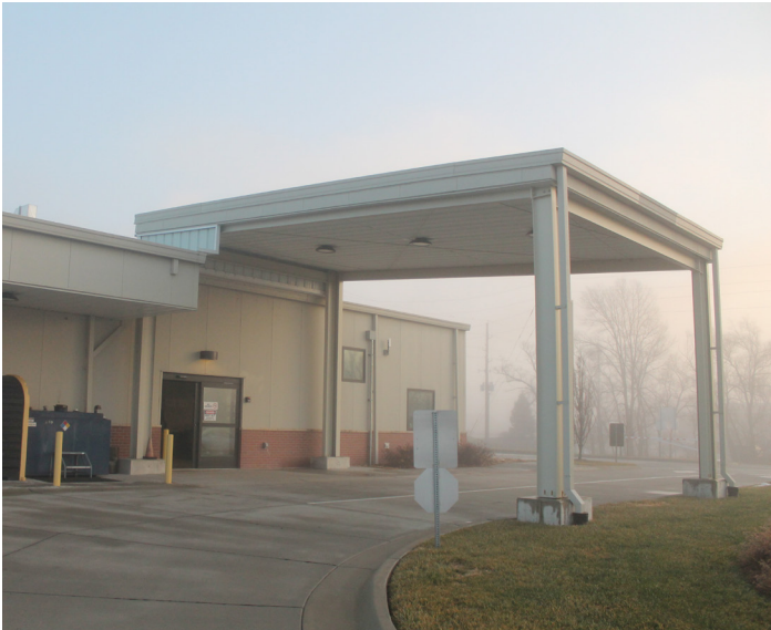
Exterior - good condition
