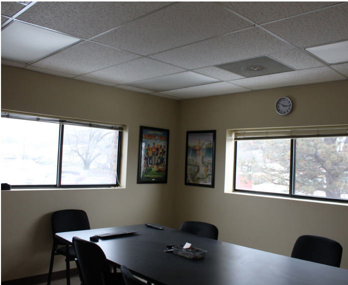
Linoleum flooring, painted gypsum board walls, ACT ceiling, good condition
