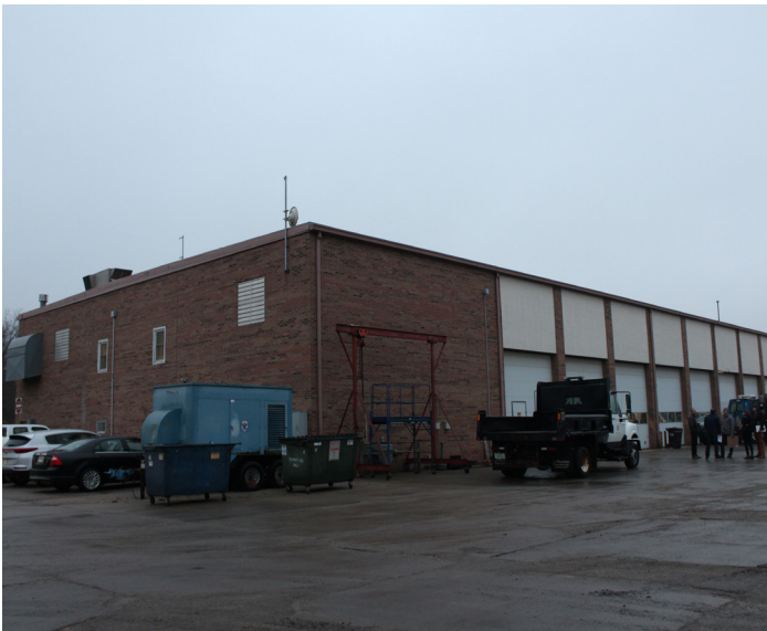
Exterior - good condition
