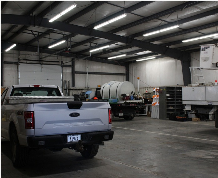
Concrete floor, pre-engineered metal structure, good condition
