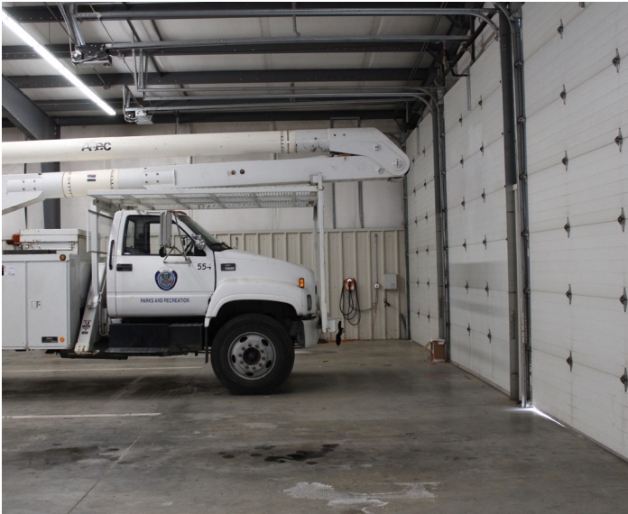
Concrete floor, pre-engineered metal structure, good condition
