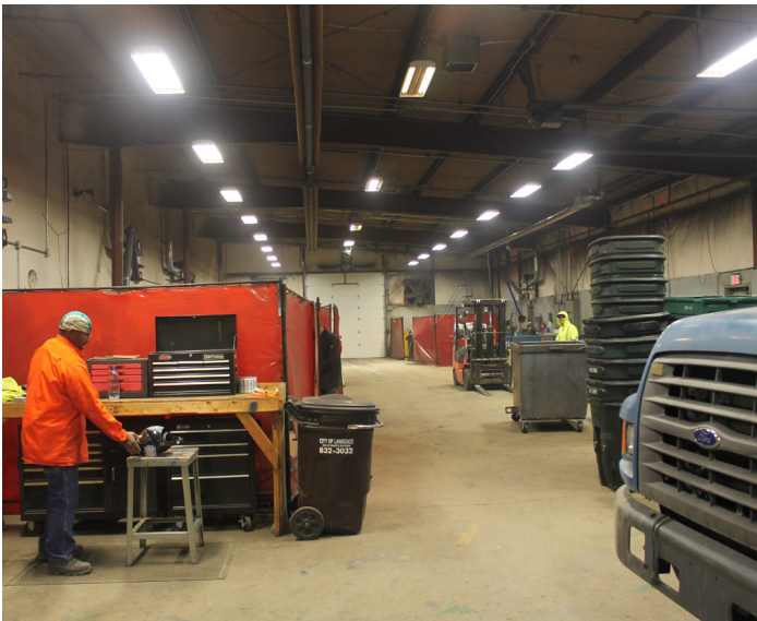
Concrete floor, pre-engineered steel structure
