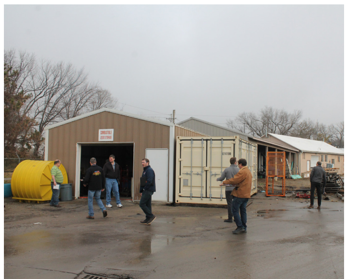
Exterior storage shed, good condition
