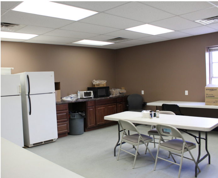
Concrete floor, painted gypsum board walls, ACT ceiling, good condition
