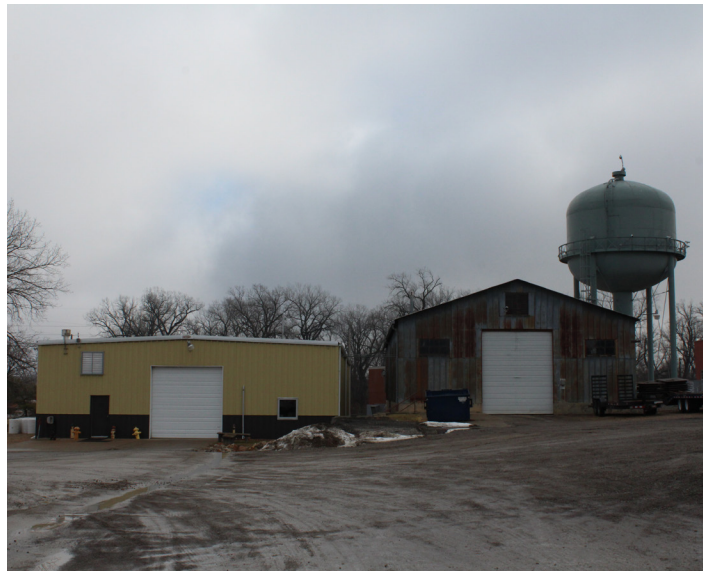
Exterior - fair condition (left) poor condition (right)
