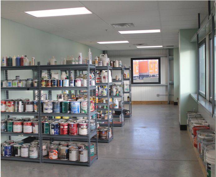
Concrete floor, painted gypsum board walls, ACT tile ceiling, good condition
