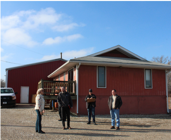
Exterior - fair condition
