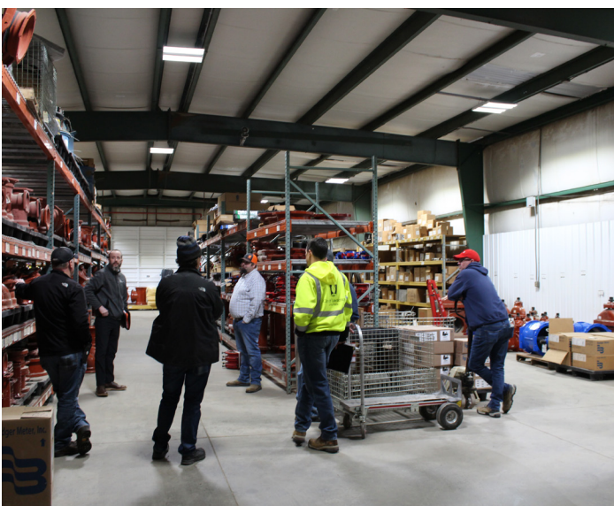
Concrete floor, pre-engineered steel structure, bag insulation, fair condition
