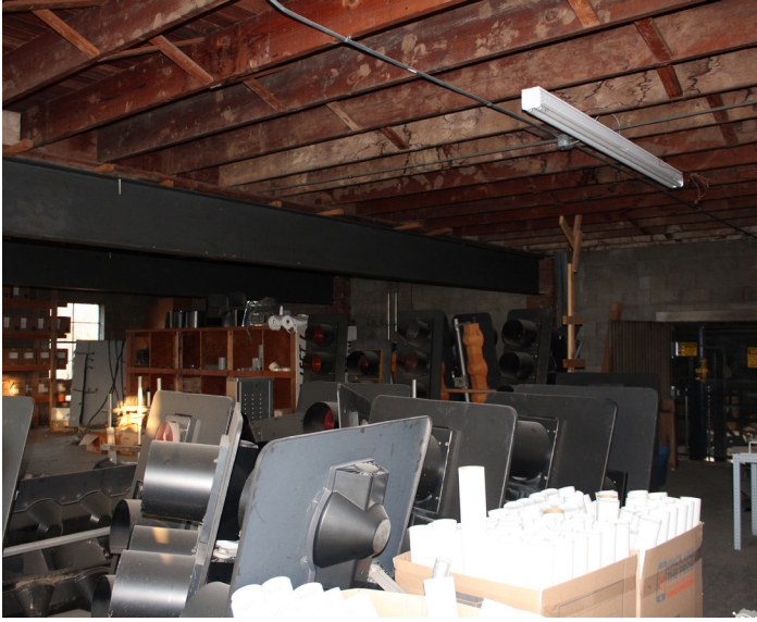
Concrete floor, CMU walls, exposed structure, fair condition
