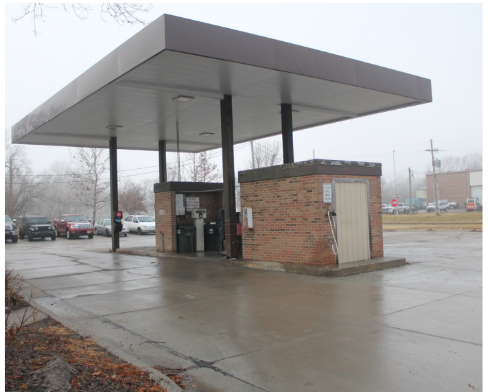
Fueling station, good condition
