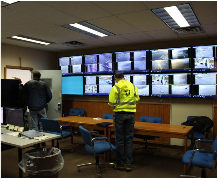
Carpet floor, painted CMU walls, decorative wood wall panel, ACT ceiling, poor condition
