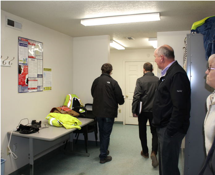
Linoleum flooring, gypsum board walls, popcorn ceiling, surface mounted fixtures,
