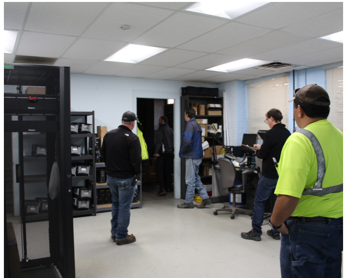
Linoleum flooring, painted CMU walls, ACT ceiling, fair condition
