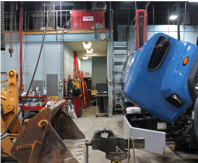
Concrete floor; painted CMU walls, exposed steel structure , fair condition
