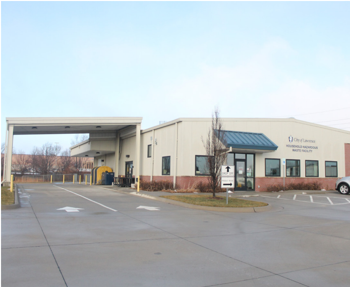
Exterior - good condition
