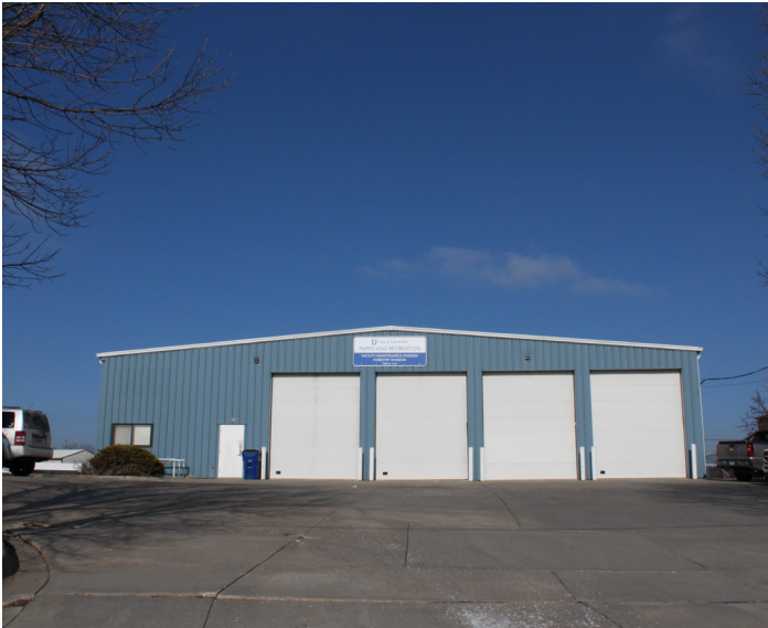
Exterior - good condition
