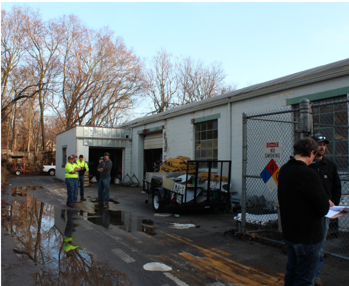
Exterior - poor condition
