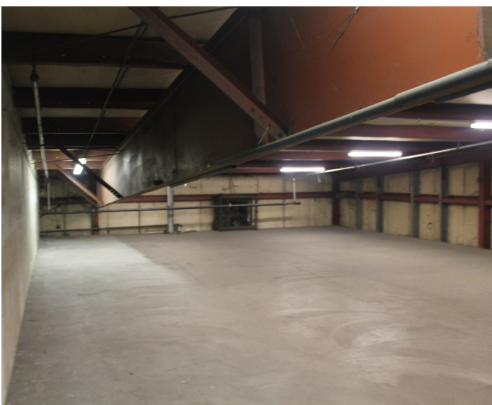
Concrete floors, pre-engineered steel structure, fair
