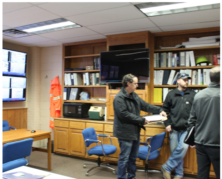
Linoleum flooring, painted CMU walls built in storage, ACT ceiling, poor condition
