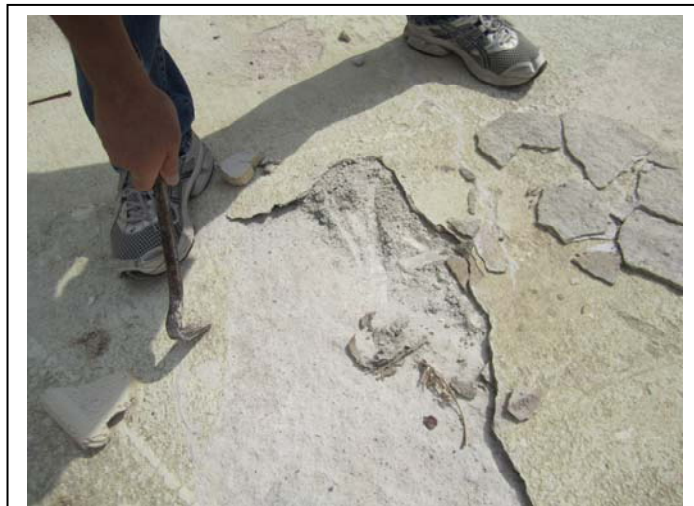
Item #6: Basin's Base Slab
