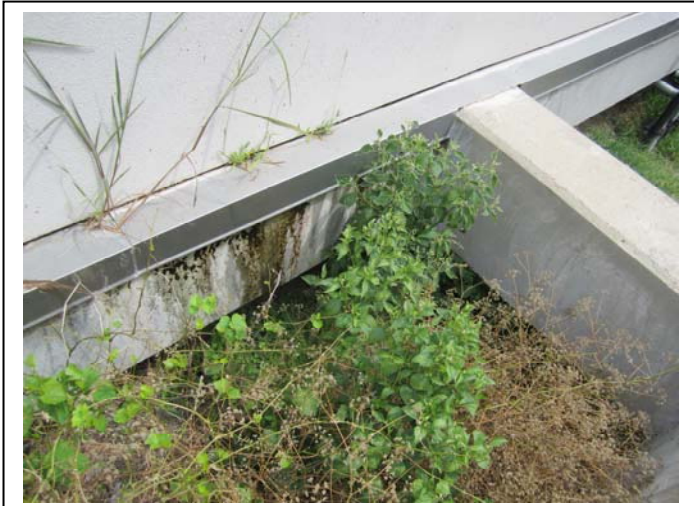
Item #5: Wall of Primary Basin's Trough
