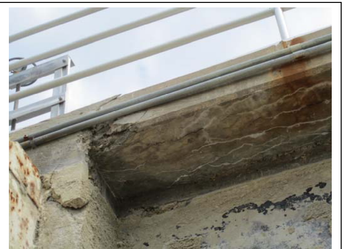
Item #4: Basin walkway near the weir troughs.
