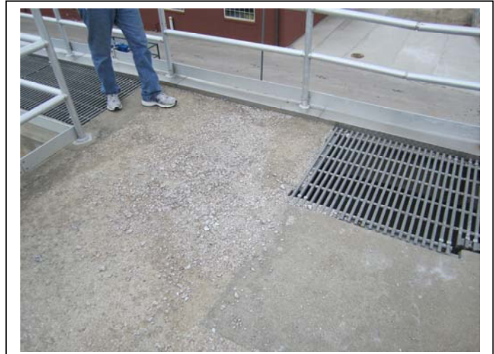
Item #2: Concrete Walkway's at Both Basins
