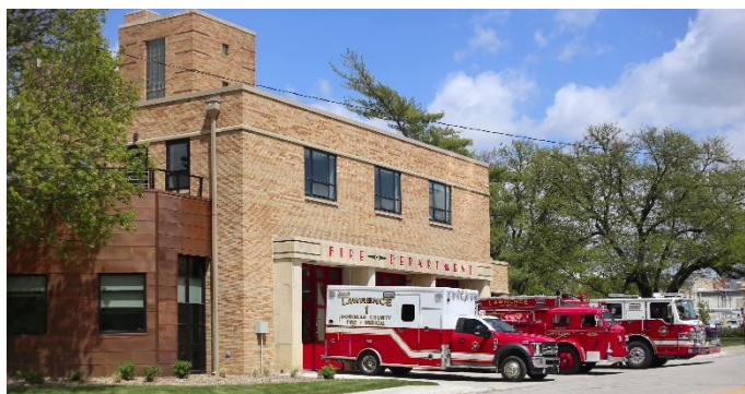
Fire Medical Station 1
