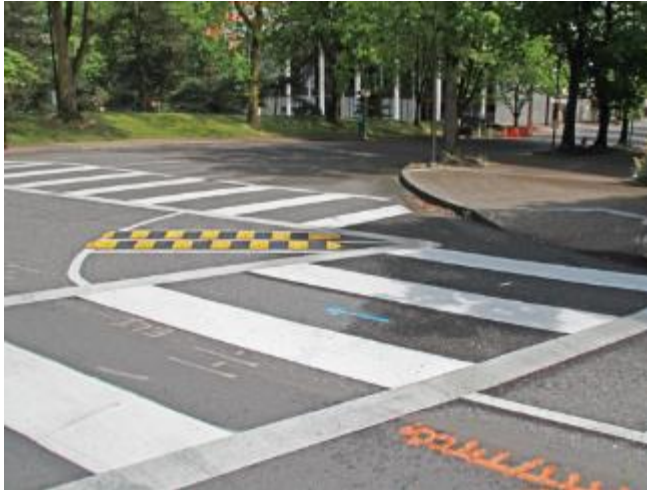
Figure 6-3: Corner Extension using Speed Humps (Source: Google)
