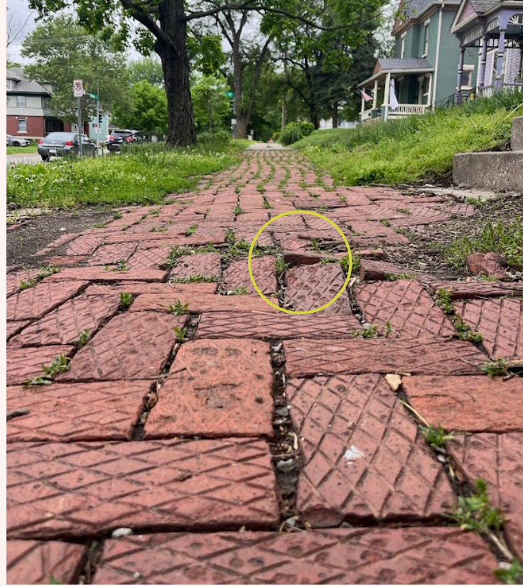
Category 2 – The sidewalk has vertical separations
