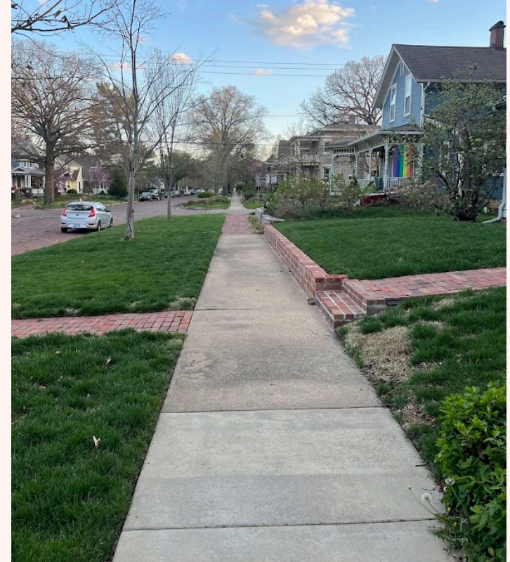
Category 6 – Accessible sidewalk
