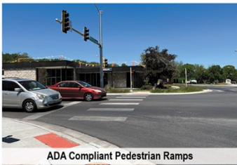
ADA Compliant Pedestrian Ramps
