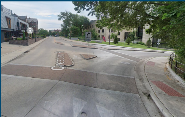
Intersection of Naismith Dr and Crescent Rd
