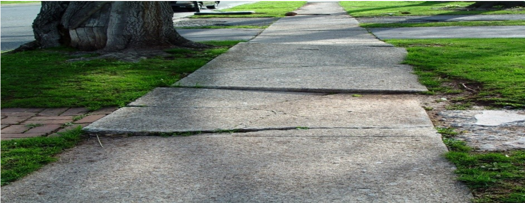
Figure 9: Sidewalk Category 2: the sidewalk has vertical separation.
