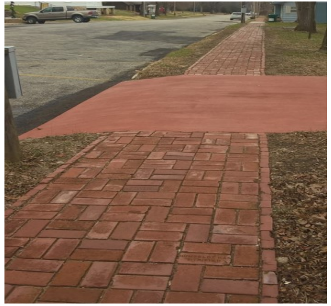
Figure 18: Brick sidewalk in good condition.
