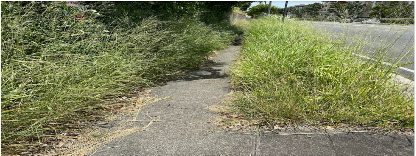
Figure 16: Sidewalk with overgrown landscape blocking the path of travel
