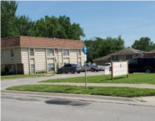
Figure 22: A bus stop without an accessible boarding pad.
