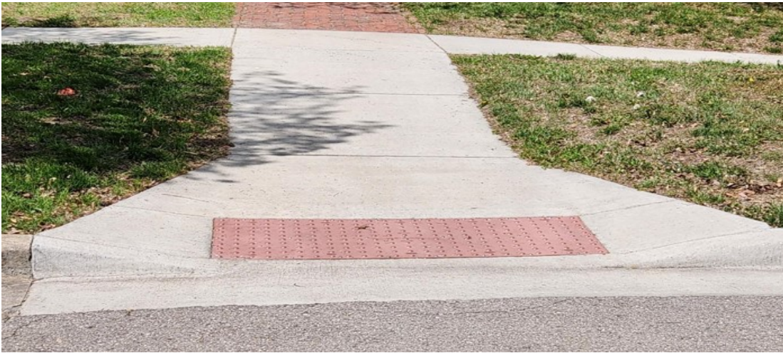
Figure 7: Category 6: a newly constructed, fully ADA-compliant curb ramp
