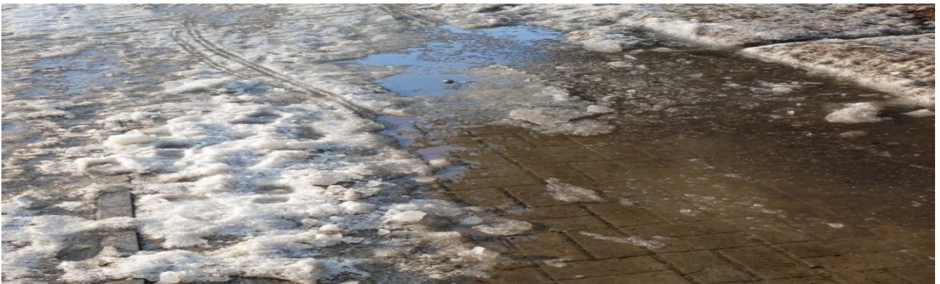
Figure 17: Sidewalk with snow and ice build-up.
