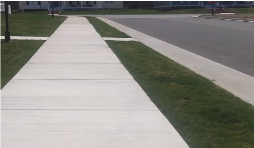
Figure 12: Sidewalk Category 6: a newly constructed ADA-compliant sidewalk.
